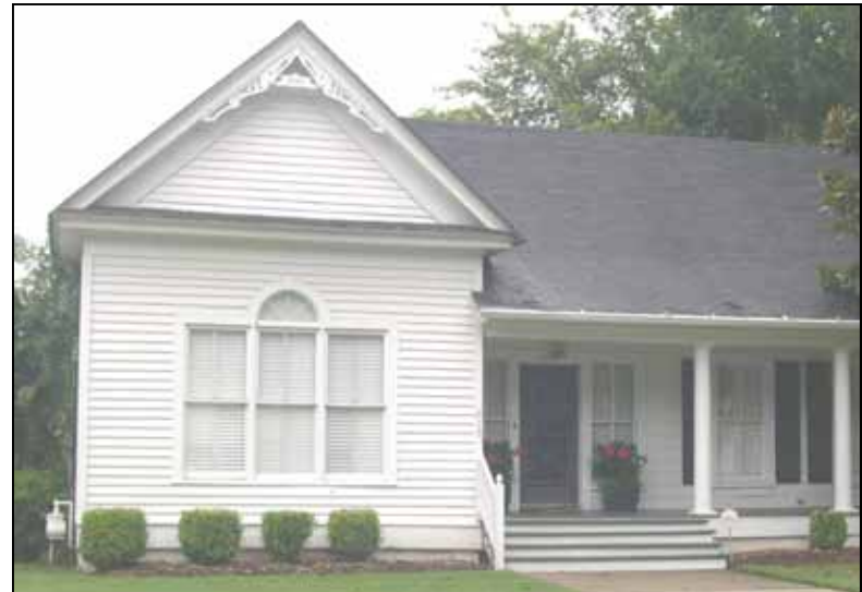
The steps of this Free Classic Queen Anne style house at 213 North Bolivar Avenue are appropriately constructed of wood.
