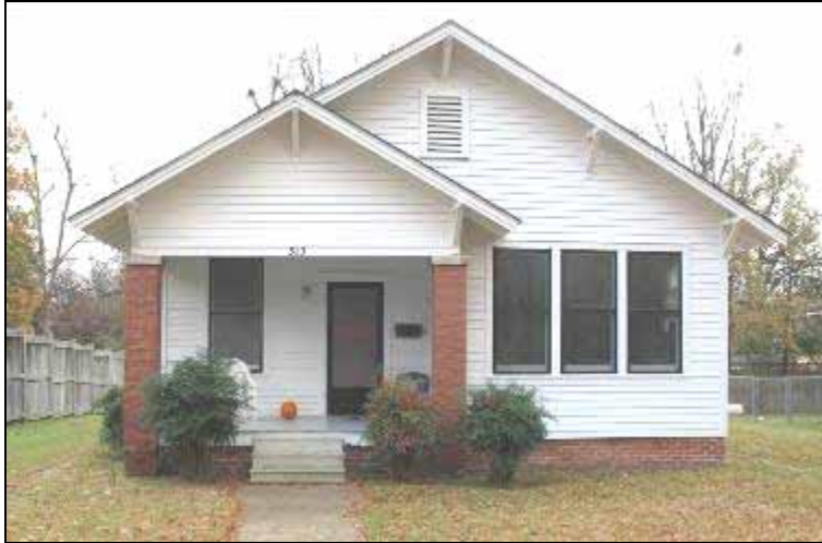
This Craftsman house at 313 South Bolivar Avenue has a projecting porch supported by brick columns typical of that style.
