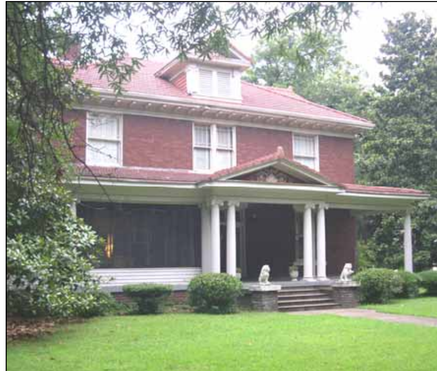
208 South Pearman Avenue features a hipped roof over the house and porch with the use of clay tile. The roof shape and material are typical of the Colonial Revival style.
