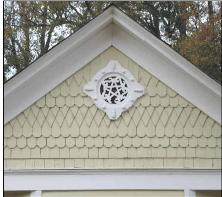
The gable at 204 South Bolivar Avenue uses a combination of wood shingle siding patterns with square, diamond, and Fish Scale to add visual interest to the gable.
