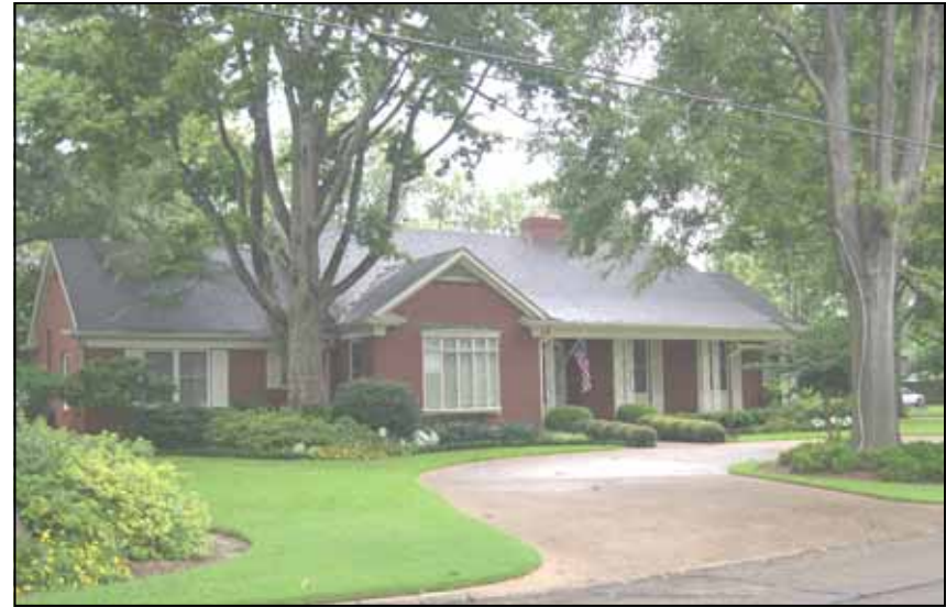
The Sledge house at 315 South Leflore Avenue was designed in the Ranch style with classical details by Greenville architect Harold Kaplan.
