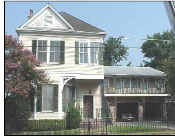
This side addition is inappropriate in proportion and scale, height, materials, massing, and roof shape. The upper and lower porches, the entrance door, and the second-story windows of this historic house have also been remodeled.
