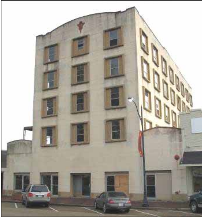
The original brick exterior of the Grover Hotel in downtown Cleveland was covered with stucco and scored to look like large blocks.
