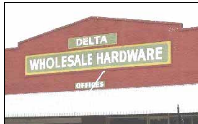
The sign on this building in Cleveland is painted in the sign board area which is delineated by a projecting brick border.
