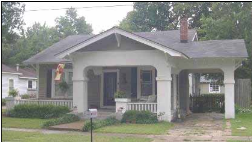
The Craftsman style house at 109 North Victoria Avenue features multiple low-pitched gable roofs with exposed rafter tips.
