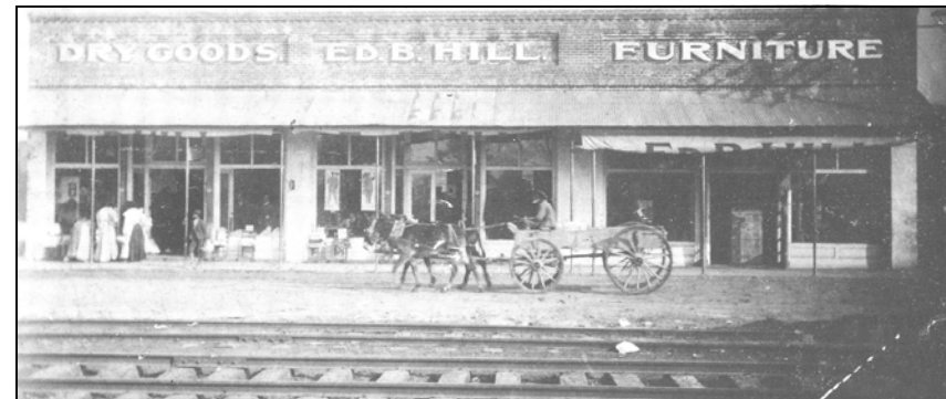
This photo of the Ed B. Hill store from the early 1900s shows a typical Cleveland storefront of the time with wide openings for glass and doors to showcase the merchandise and light the interior. Photo from Cleveland: A Centennial History.
