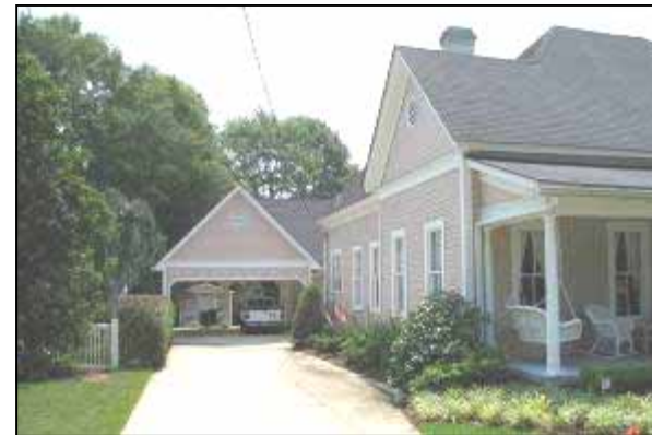
This example of a carport addition is very successful as it does not compete with the historic house and uses similar materials and roof pitch to maximize the compatibility.
