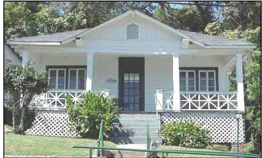
The lattice used to enclose the crawl space beneath this historic house in Natchez is an example of an inappropriately installed enclosure as it overlaps and obscures the brick supporting piers.
