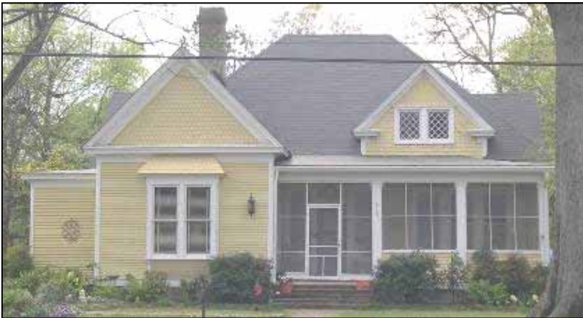
204 South Bolivar Avenue is an excellent example of the Queen Anne style as it retains many original features including: wood double hung sash windows, wood lap siding, shingle siding in the gables, and a multi-gable and hip roof.
