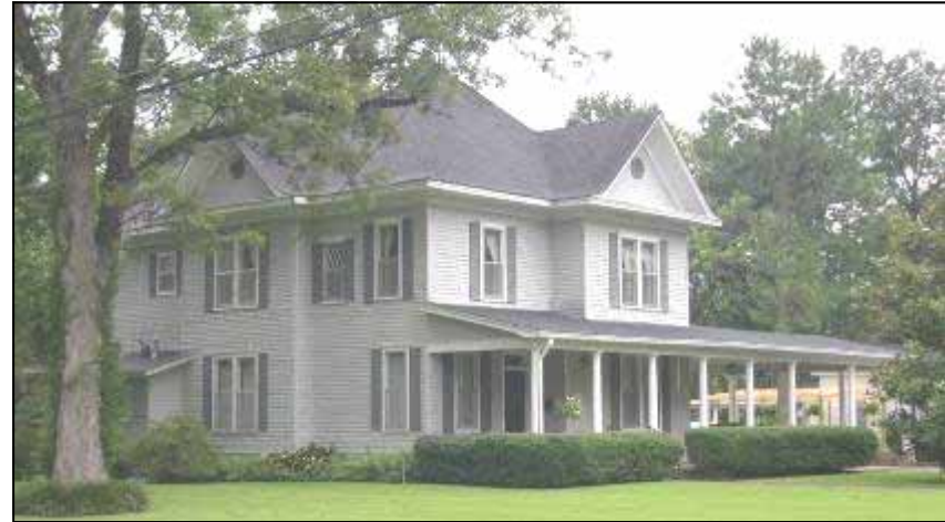
301 South Bolivar Avenue has Queen Anne massing and a porch with Tuscan columns characteristic of the Free Classic Queen Anne style. The original wrap around porch has been altered to the current porch but also had Tuscan columns.
