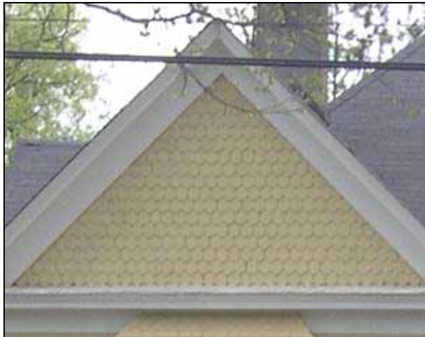
212 South Bolivar Avenue uses a rounded shingle siding in the gable, commonly known as a Fish Scale pattern.
