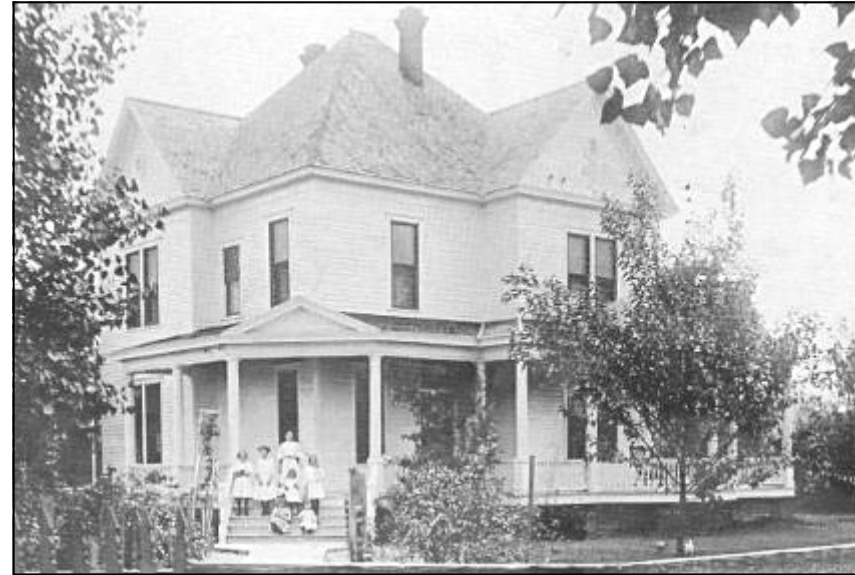
The E.J. Nott house at 301 South Bolivar pictured circa 1904 still survives to this day although the porch has been altered. Photo from Reflections of Bolivar County.
