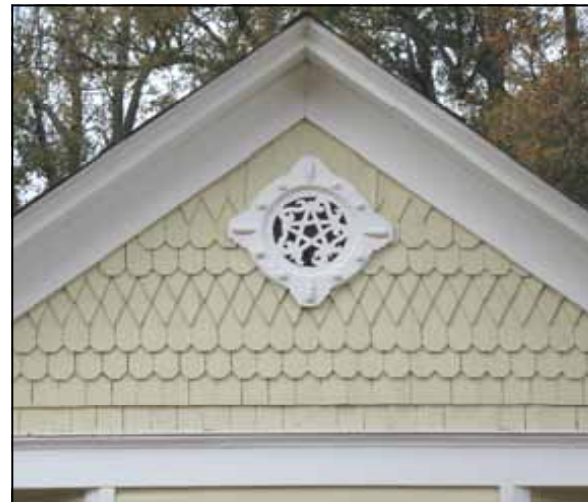
The gable at 204 South Bolivar Avenue features a combination of wood shingle siding patterns with square, diamond, and Fish Scale typical of the Queen Anne style of architecture.
