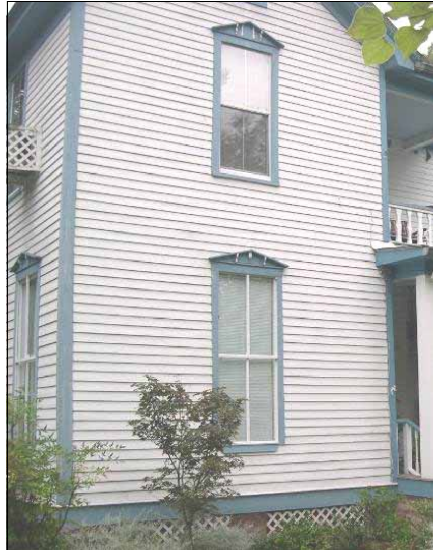
This Folk Victorian style house at 214 South Bolivar Avenue retains its original horizontal wood lap siding.
