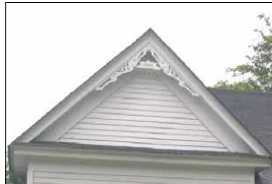
The gable at 213 North Bolivar Avenue features a decorative vergeboard or bargeboard in the upper portion of the gable made up of cut pieces of wood to form a pattern.
