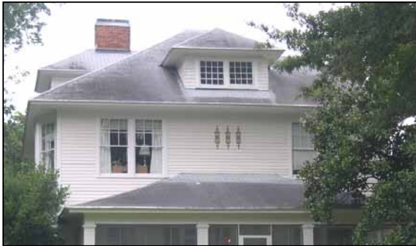
200 South Pearman Avenue has a dormer with a hipped roof matching the main roof and windows to light the attic space under the roof.
