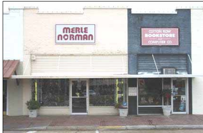
These buildings on Sharpe Avenue show the correct installation and projection for suspended canopies on a commercial building. The projecting flat canopies are anchored by rods which is typical of commercial buildings built from the 1920s to 1940s.
