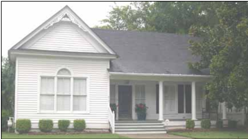
The house at 213 North Bolivar Avenue exhibits Queen Anne massing with Colonial Revival details such as Tuscan Columns and a Palladian window unit in the front bay.
