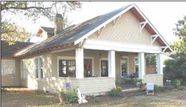
The Craftsman style house at 115 North Leflore Avenue has full width undercut porch supported by wood box columns and a half wall balustrade.
