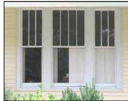
The three-over-one and four-over-one windows on the left are typical windows found on Craftsman style houses.
