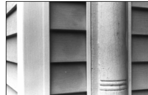
Examples of vinyl siding showing the installation of J-channels around every opening and the historic trim, if it survived the installation process.
