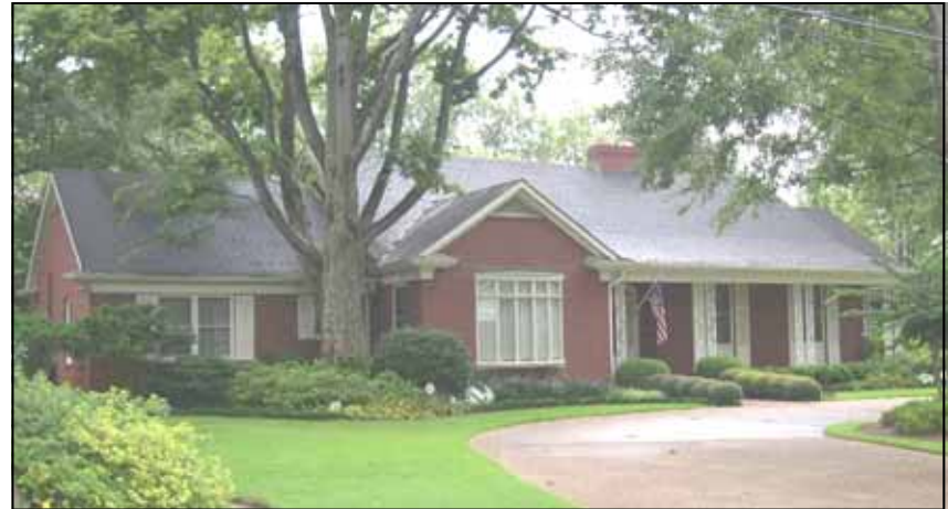
315 South Leflore Avenue
