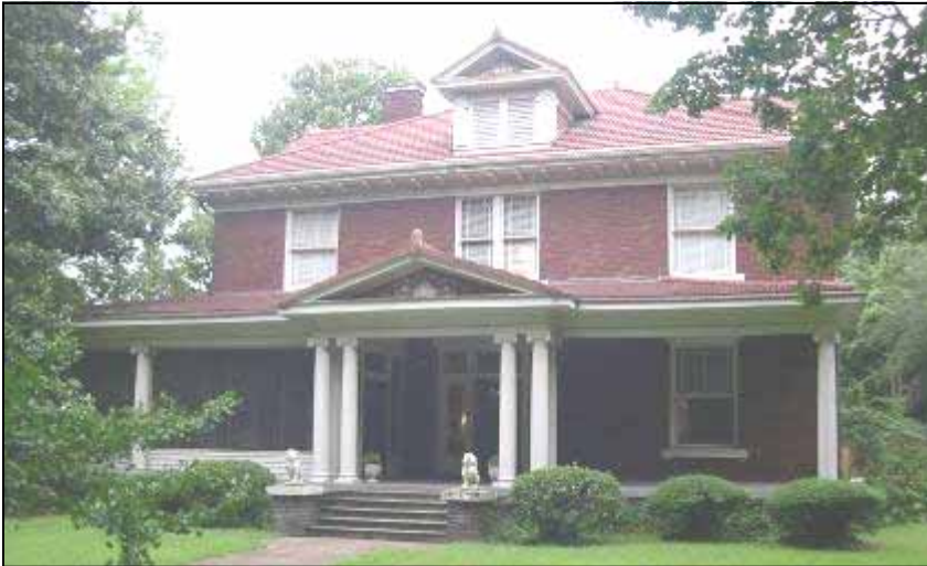
This Colonial Revival House at 208 South Pearman Avenue features a full width porch with Ionic columns and paired columns at the entrance typical of that style of house.
