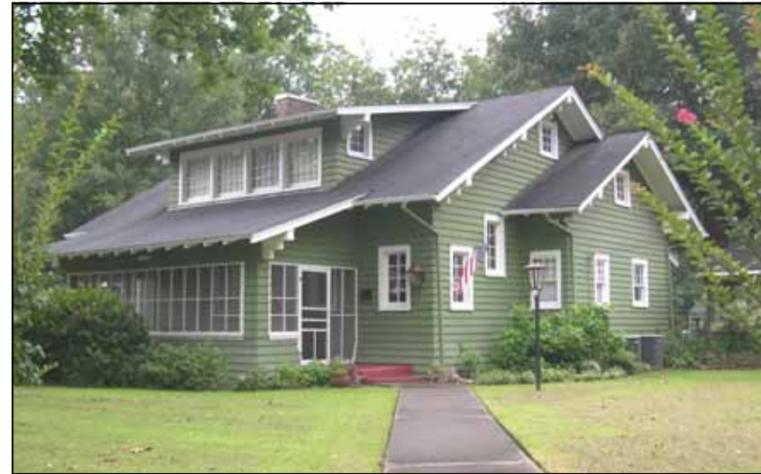
500 South Leflore Avenue
