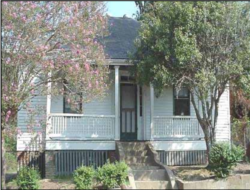
This vernacular house in Natchez features a crawl space appropriately enclosed with vertical boards nailed to a frame between the brick piers.
