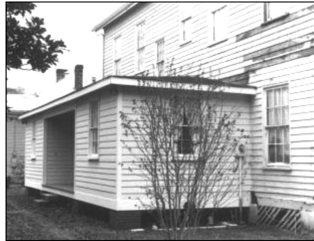
This rear addition is secondary to the original house and reads as an addition yet uses materials similar to the original house.
