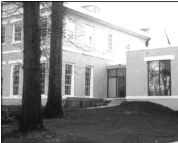
This National Park Service photograph illustrates an appropriate design for a modern addition and a proper method of connecting it to the historic building.
