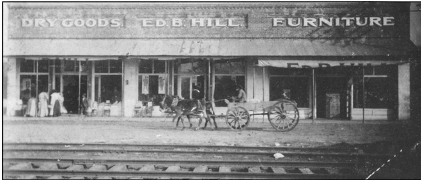
The Ed B. Hill Store pictured from the early 1900s was an early brick commercial building in Cleveland near the railroad tracks. Photo from Cleveland: A Centennial History.
