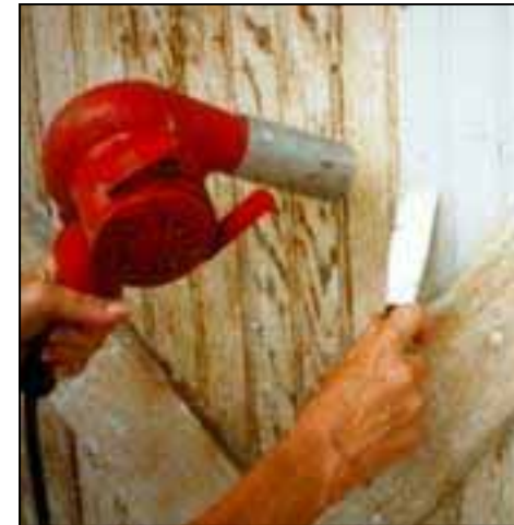
These National Park Service photographs illustrate a painted finish with severe peeling (left) and the use of a electric heat gun (right) to remove a deteriorated paint finish.
