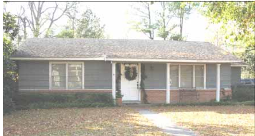
The Ranch style house 117 North Leflore Avenue has a small overhang that acts as a front porch and is supported by columns on a concrete deck.
