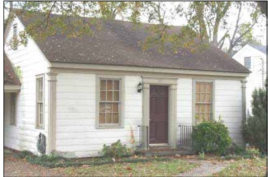
505 South Leflore Avenue
